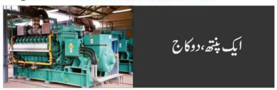
Steam is very powerful. It does not only run an engine but also possesses the ability of air conditioning besides its various other uses. Diesel and/or gas generators not only produce electrical power but may also produce steam which may be used for heating or cooling. This is like killing many birds with one stone. Technically, this is known as Co-generation.
