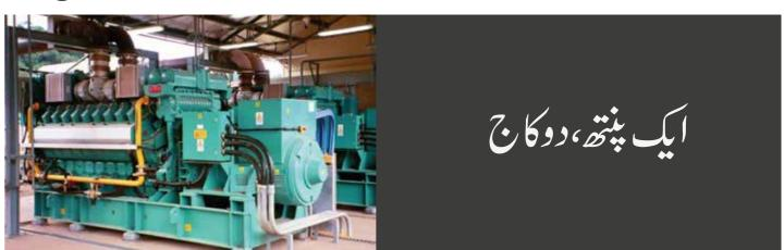
Steam is very powerful. It does not only run an engine but also possesses the ability of air conditioning besides its various other uses. Diesel and/or gas generators not only produce electrical power but may also produce steam which may be used for heating or cooling. This is like killing many birds with one stone. Technically, this is known as Co-generation.
