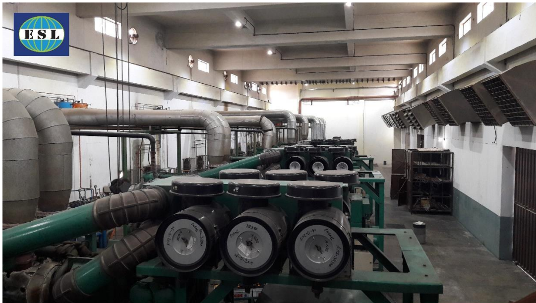
GENERATOR ROOM / POWER PLANT VENTILATION
