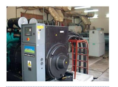
ESL supplied, installed and commissioned 1 x 1410 kVA Aksa DG set to the Hospital. Has also provided synchronizing systems for all 3x1410 KVA diesel, 1x1370 KW Cummins gas and 1x 1600 KW CAT gensets. Has done upgradation of LT distribution panels and Medium voltage substation. ESL has completed this project in record time of six weeks without any shutdown to the main hospital building.
