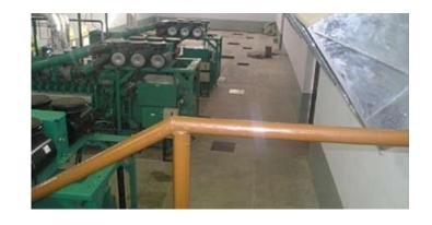
ESL supplied, installed and commissioned 2 x 1.2 MW Gensets and synchronized them with existing 6 x 1.2 CPG Gensets at 11 kV.
