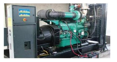
ESL supplied 5 x 2250 kVA Aksa Gensets and synchronized them with existing 2 x 1250 kVA Cummins and 1 x 500 kVA CAT gensets.
