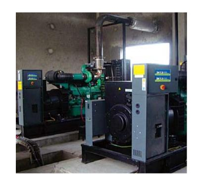
ESL supplied, installed and commissioned 1 x 1675 kVA genset and synchronized it with existing 3 x 1000 kVA DG sets. Has also provided uninterrupted load transfer facility between three WAPDA transformers and gensets. ESL supplied, installed and commissioned 1 x 1675 kVA Genset, 1 x 1130 KVA Genset and synchronized them with very old 2x 1000 KVA gensets. Has also provided uninterrupted load transfer facility between three WAPDA transformers and gensets at Jehlum Plant.
