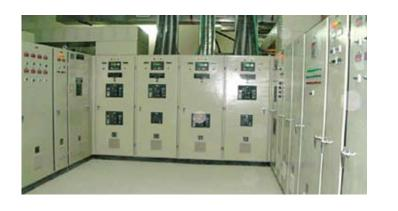
ESL supplied, installed and commissioned 2 x 825 kVA Gensets and synchronized them with existing 1 x 500 kVA Genset involving uninterrupted load transfer facility between two Wapda transformers and gensets to Hattar Plant.
