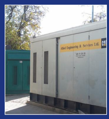
ESL synchronized 1 x 635 kVA Caterpillar, 1 x 725 kVA Caterpillar and 1 x 681 kVA Cummins Diesel Gensets in Mobilink, Islamabad. This allows the Customer to free 1 x 400 KVA genset from their operations, which results in considerable savings. The job has been
