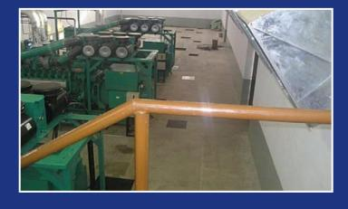
ESL supplied, installed and commissioned 2 x 1.2 MW Gensets and synchronized them with existing 6 x 1.2 CPG Gensets at 11 kV.
