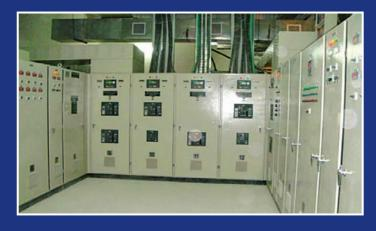
ESL supplied, installed and commissioned 2 x 825 kVA Gensets and synchronized them with existing 1 x 500 kVA Genset involving uninterrupted load transfer facility between two Wapda transformers and gensets to Hattar Plant.
