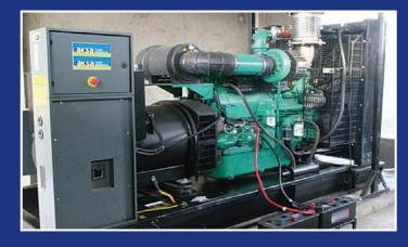
ESL supplied 5 x 2250 kVA Gensets and synchronized them with existing 2 x 1250 kVA Cummins and 1 x 500 kVA CAT gensets. Has also provided uninterrupted load transfer facility between five WAPDA transformers and gensets to Lahore Plant.
