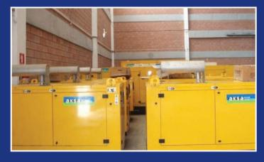
ESL supplied, installed and commissioned 100 x 30 kVA and 1 x 160 kVA Diesel Gensets. Also extending maintenance services to various branches of the bank throughout Pakistan, under the Annual Maintenance Contract.
