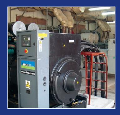
ESL supplied, installed and commissioned 1 x 1675 kVA genset and synchronized it with existing 3 x 1000 kVA DG sets. Has also provided uninterrupted load transfer facility between three WAPDA transformers and gensets to Akora plant.
